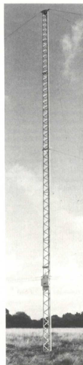
Typical lattice mast supporting HF antenna and balun.
