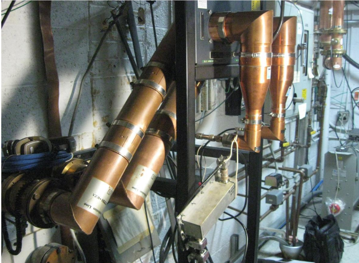
Rigid Feed Lines to the Dielectric Communications TF Series CH2 Superturnstile Antenna
