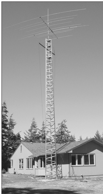
Fig 28.10 — A guyed tower with a good-sized load of antennas at XE2DV-W7ZR in Baja California, is shown at the left. At the right, the Trylon Titan self-supporting tower of W7WVF and N7YYG in Bandon, Oregon. (K7LXC photos)
