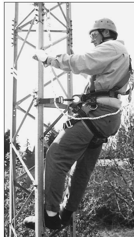
Fig 28.21 — The fall-arrest lanyard is above the climber so that the climber can climb up to it. The fall-arrest and positioning lanyards are then “leapfrogged” so that the climber remains attached to the tower 100 percent of the time. (K7LXC photos)
