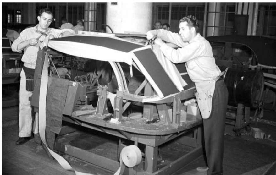
Soft trim assemblies were part of the Highland Park production schedule. Here, skilled craftsmen assembly a late-1940s Ford convertible top.
