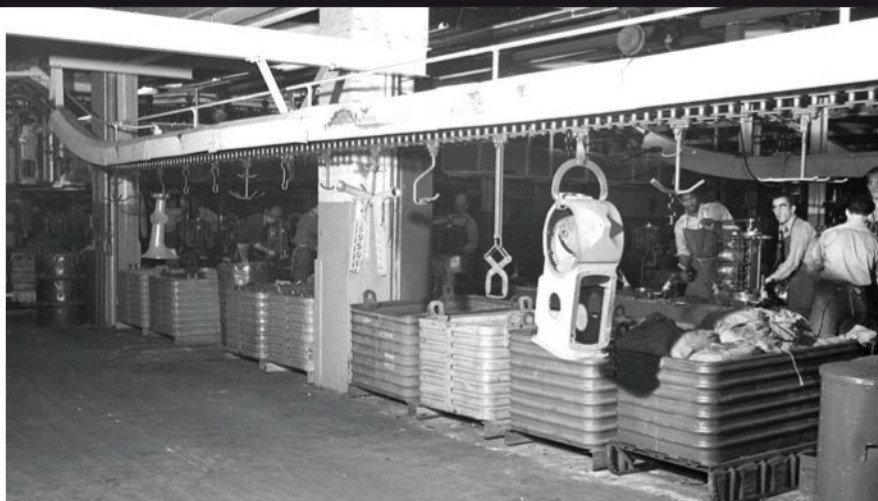
Assembly line techniques were honed by Ford at the Highland Park plant, illustrated here with major components for the 2N tractor being delivered via conveyor system.
