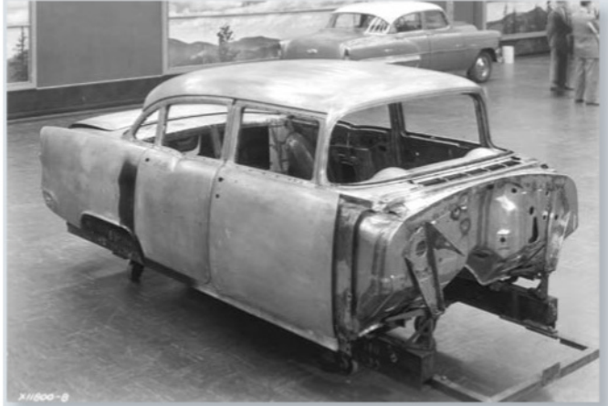
An early sample body from Fisher Body is shown here inside the Argonaut Building's 11th floor auditorium. Early bodies and chassis were combined for testing at GM's Milford, Mich., proving grounds. Deliveries of early bodies began in February 1954. (GM Media Archive)
